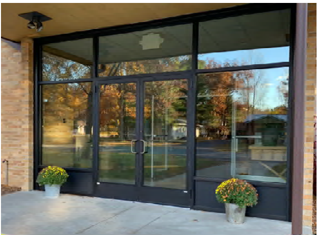
West entrance with new windows & doors!
