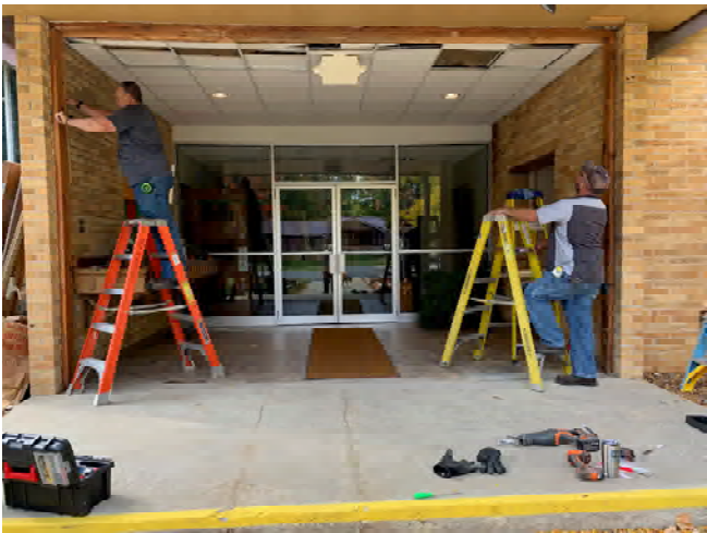
Zion's west entrance during renovation!
